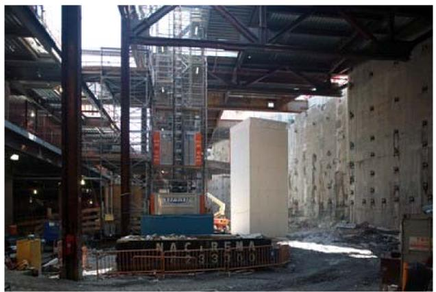
September 2009. Last Column (in climate controlled enclosure) and the exposed slurry wall.
