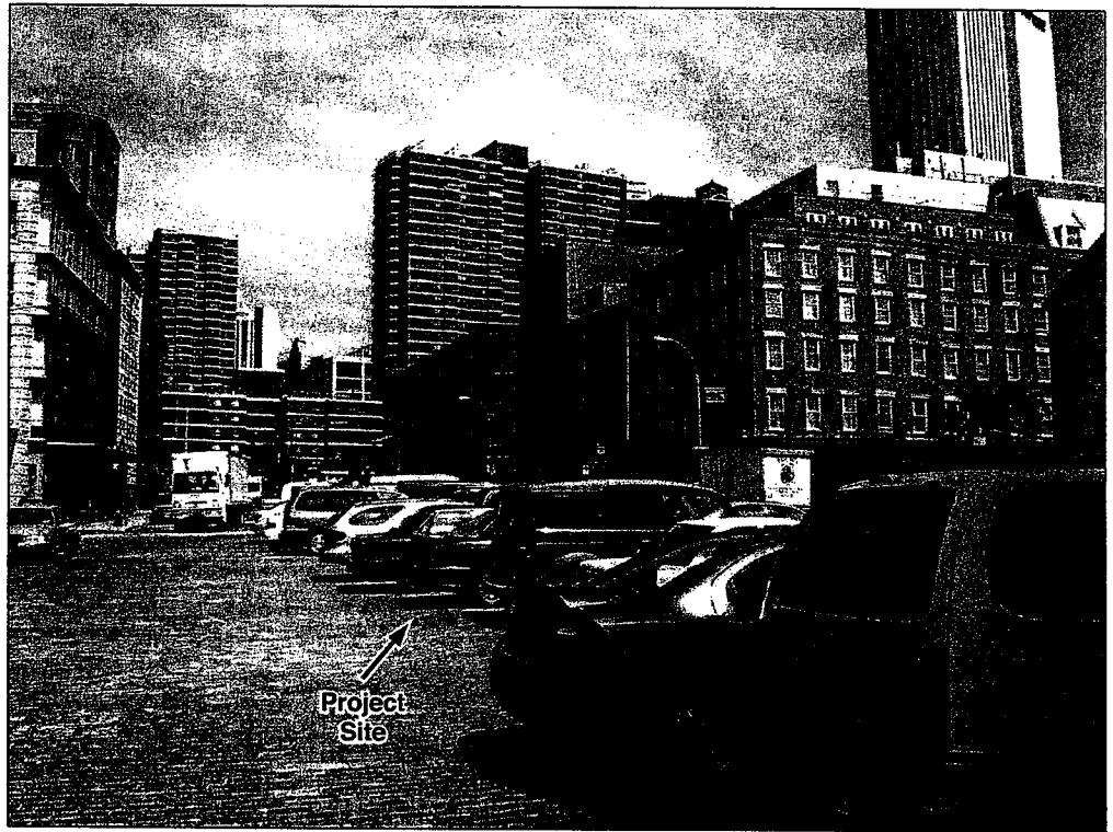
Northeast side of Peck Slip 6
