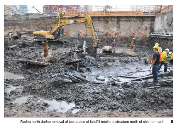
Facing north during removal of top course of landfill retaining structure north of ship remnant (in foreground). WTC slurry wall is in background and demising wall is to the right
