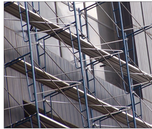
Scaffolding on the exterior of 130 Liberty Street.
