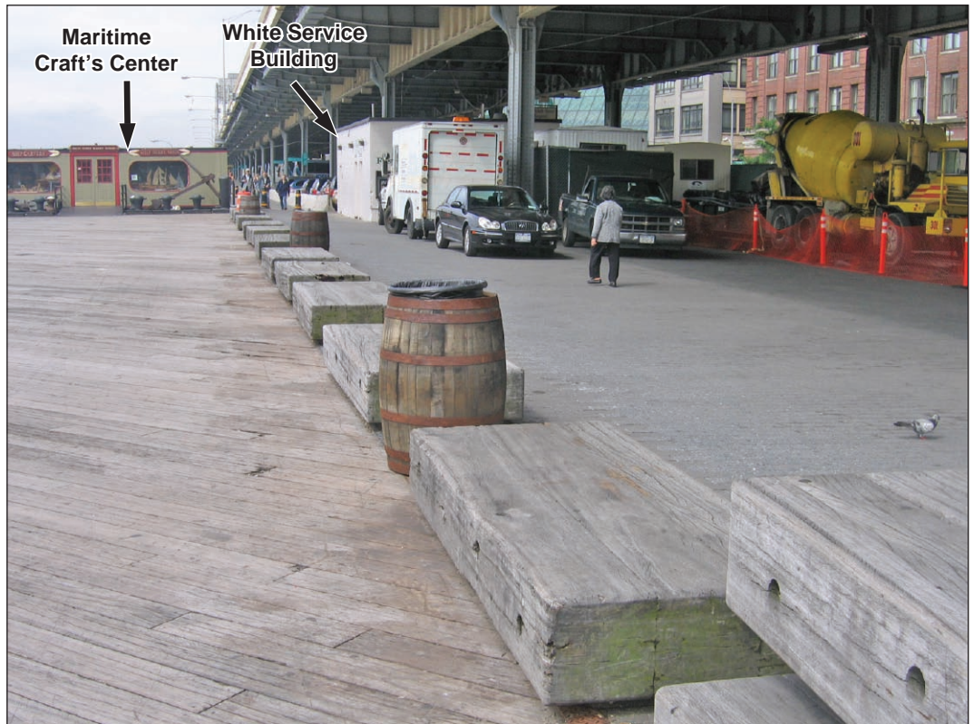
View south from near Pier 16 2
