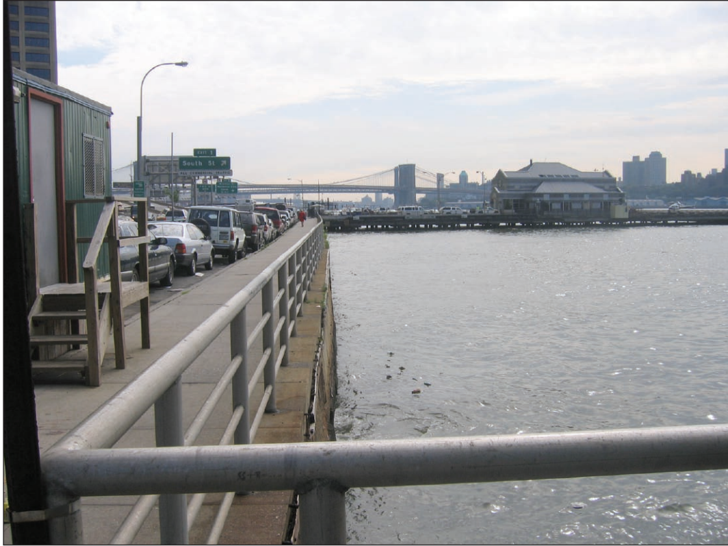
View north of the walkway/ bikeway from the Battery Maritime Building 8
